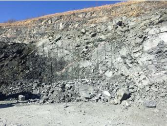
Even though some of the presplit walls were located in areas of intersecting jointing planes, the presplit held and provided a safer area below, once the walls were scaled.
